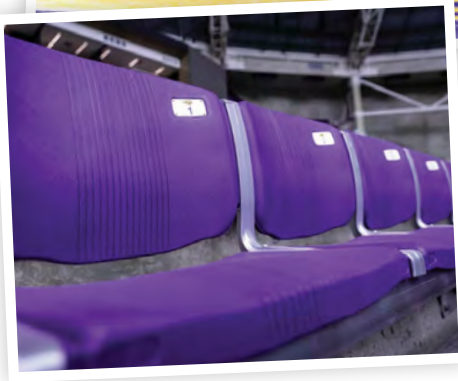
The first features of the UNI-Dome's phase two renovations were completed over the summer, adding new seating, expanded suites and other fan amenities throughout the stadium.
